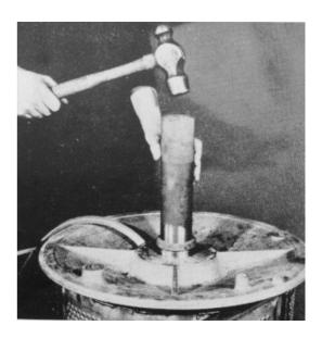
18. Fit the spacer sleeve and the circlip on the shaft. Place the spacer sleeve on the shaft's face for the rear bearing.
